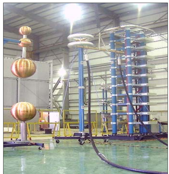
Fig. 1: Impulse voltage test generator IG 200/2000 G
