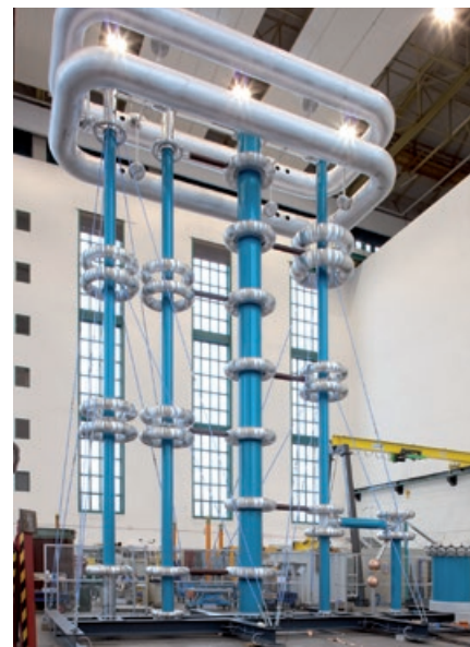
Fig. 16 Calibration of the 2000 kV DC Test System
