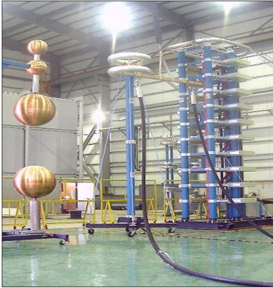
Figure 1: Impulse voltage test generator IG 200/2000 G
