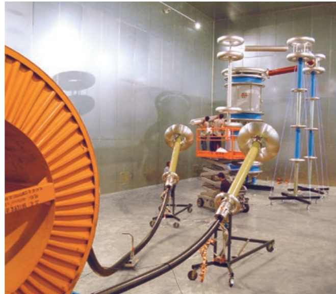
Fig. 5 Water-filled test terminations used for an AC routine test of a high voltage cable
