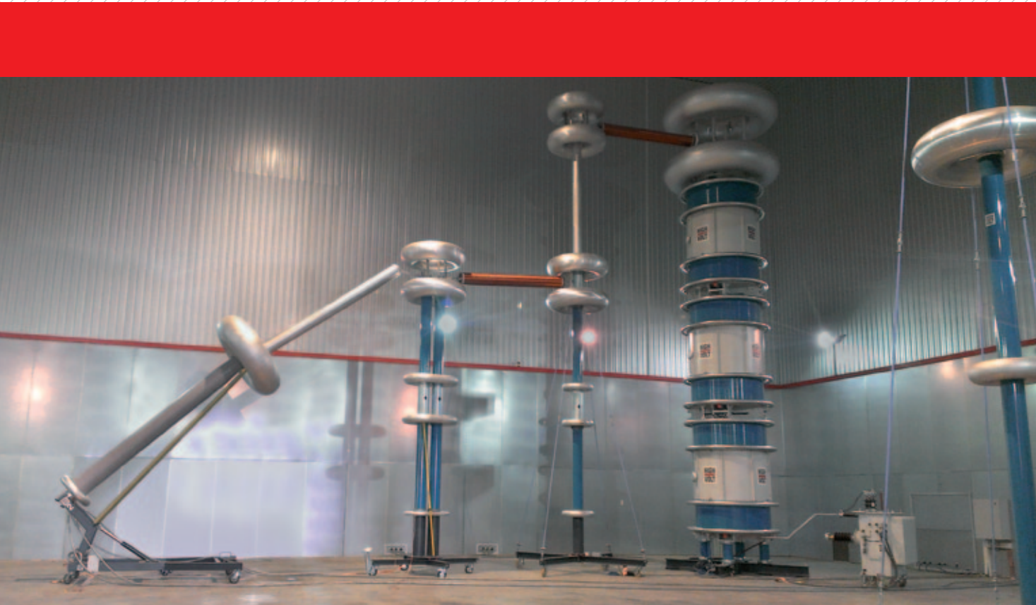
Fig. 2 Shielded room SSC 35/26/17 (incl. optional features) with integrated AC resonant test system WRM 5570/800 for type testing of high-voltage cables
